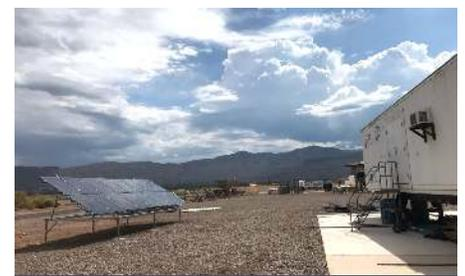
DesaliNEWT 3kW, 2gpm Pilot System
